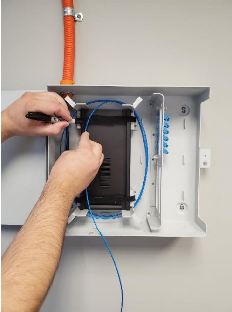
Figure 3. Coil the tube back into the panel and mark where the tube will enter the splice tray. Strip the tube at this point leaving loose fibers exposed and ready to be spliced.
